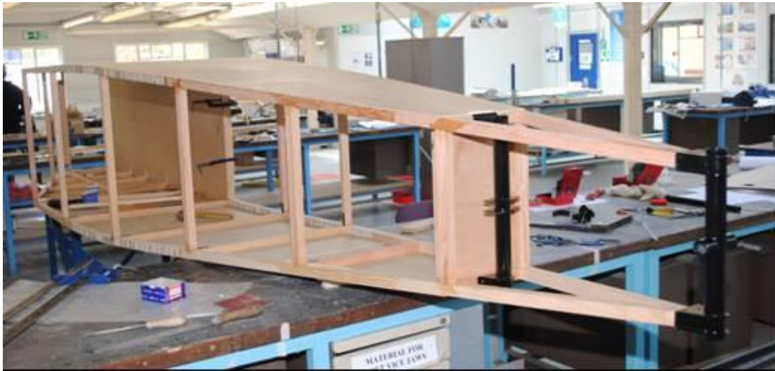
The two sides of fuselage joined with the cross members. Also the tail plane front and rear attachment fittings are shown (similar to original design).
