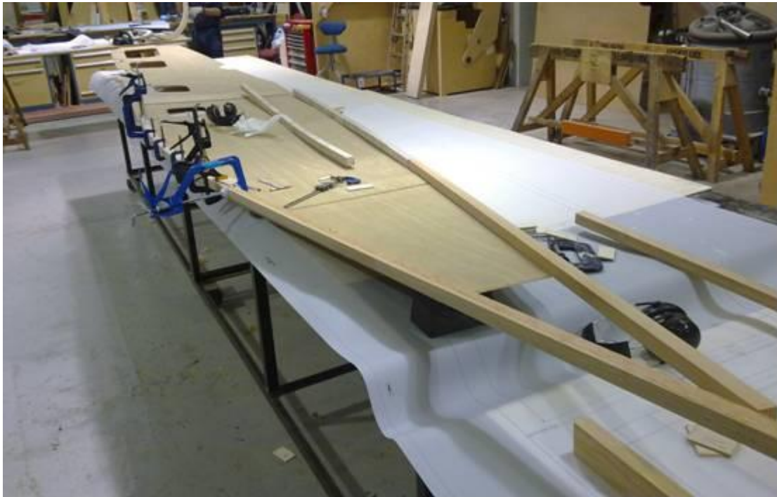
Early stages of fuselage manufacture. Each side of fuselage was cut from 3mm ply with the longerons and struts being attached to the ply. The ply provides the strength as the design was not using the original method of metal brackets/fittings and tensioned wires.
