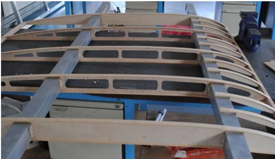
Construction of wing showing aluminium box spars, ribs and rib front packing pieces.
